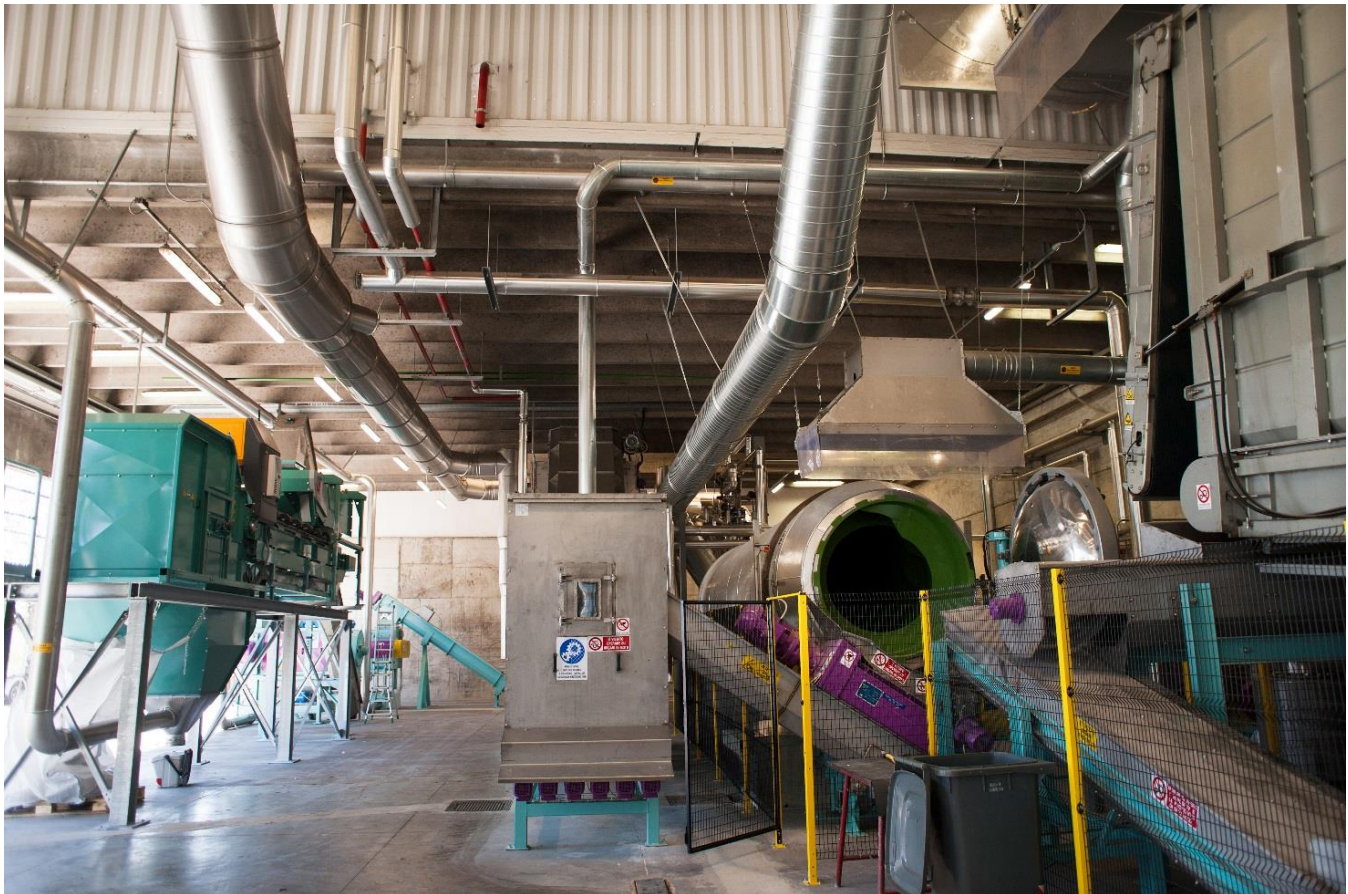
AHP waste pre-treatment plant
